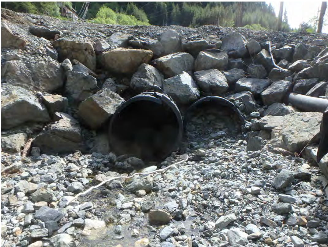
Photograph 10. West Fork Sawmill Creek twin culvert beneath hydroelectric facility access road. Note right culvert is filled with debris. Photograph taken May 31, 2016.
