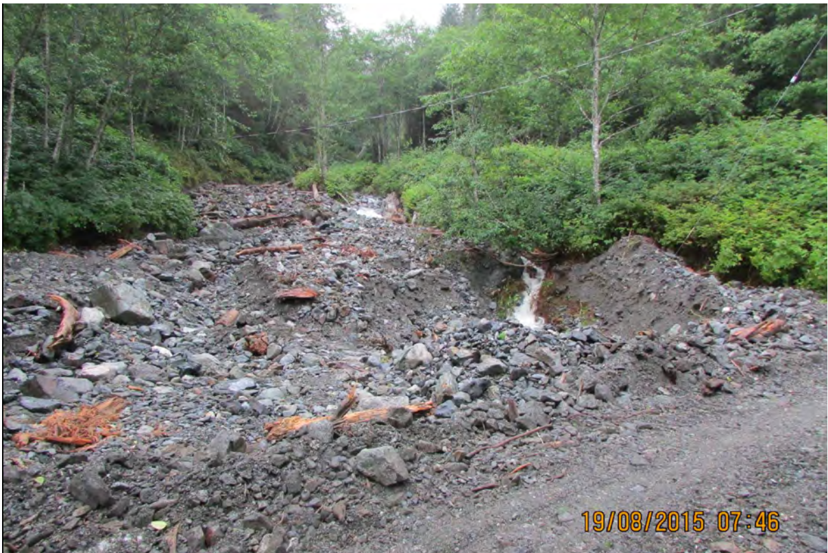
Photograph 8. West Fork Sawmill Creek channel, upstream from Blue Lake Road on August 19, 2015. Photograph provided by CBS
