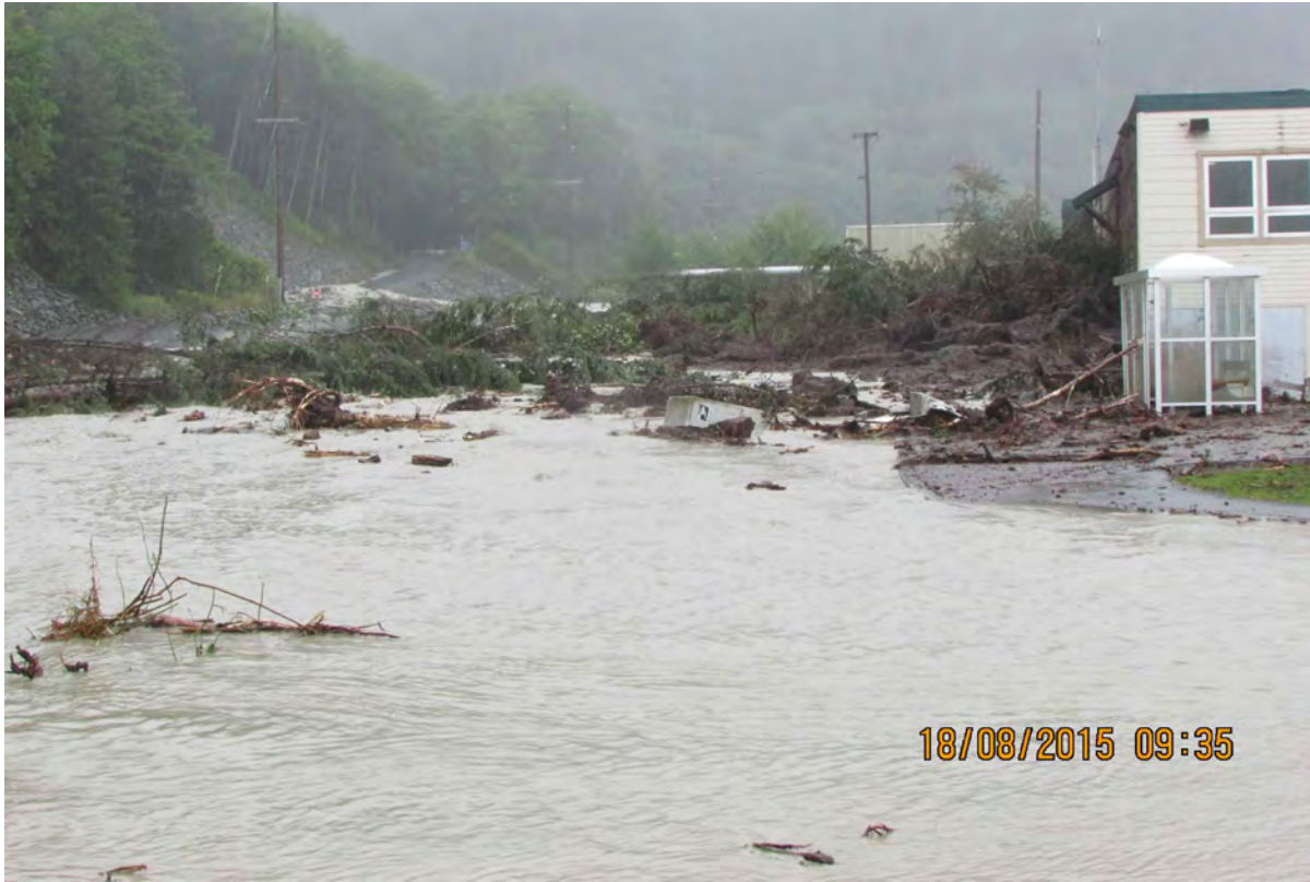
Photograph 1. Debris against administration building on August 18, 2015. Photograph provided by CBS
