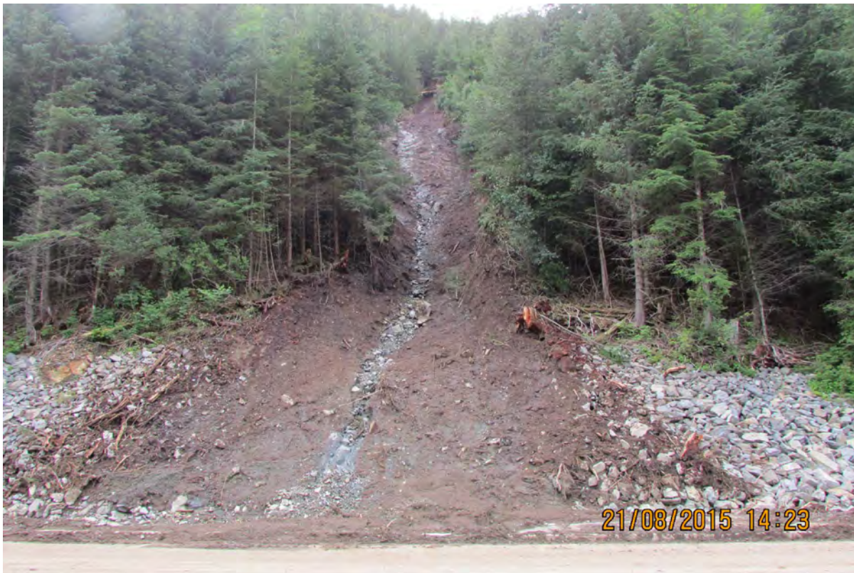
Photograph 2. Sawmill Creek Road debris flow on August 21, 2015. Photograph provided by CBS
