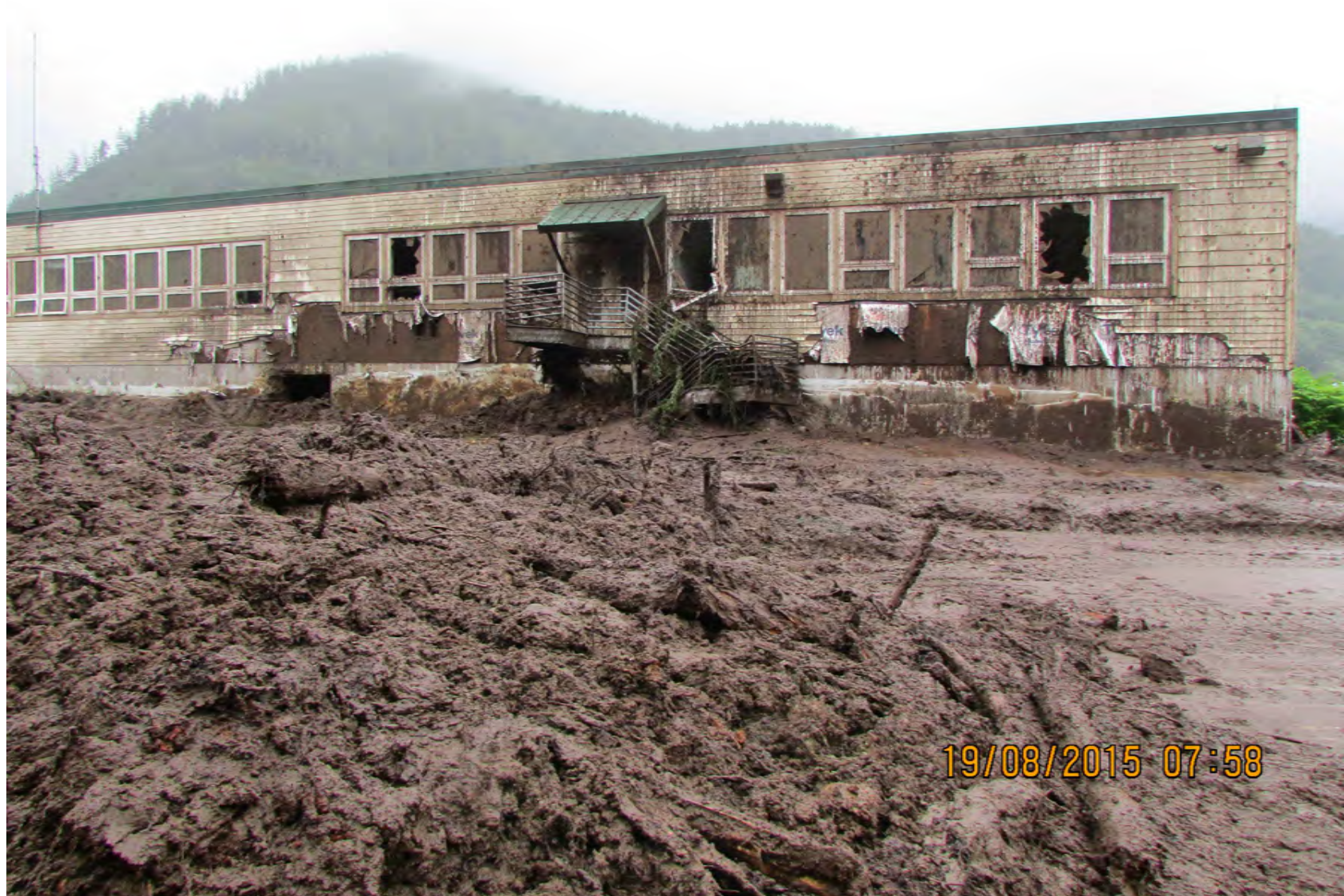
Photograph 3. Damage to Administration Building from Sawmill Creek Road debris flow. Photograph provided by CBS
