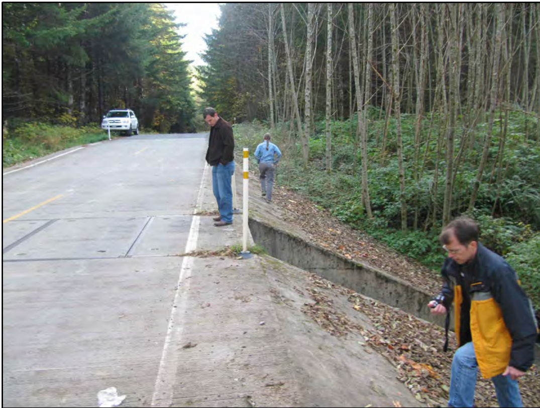
Photograph 20. Vented ford with removable concrete cover over box culvert.
