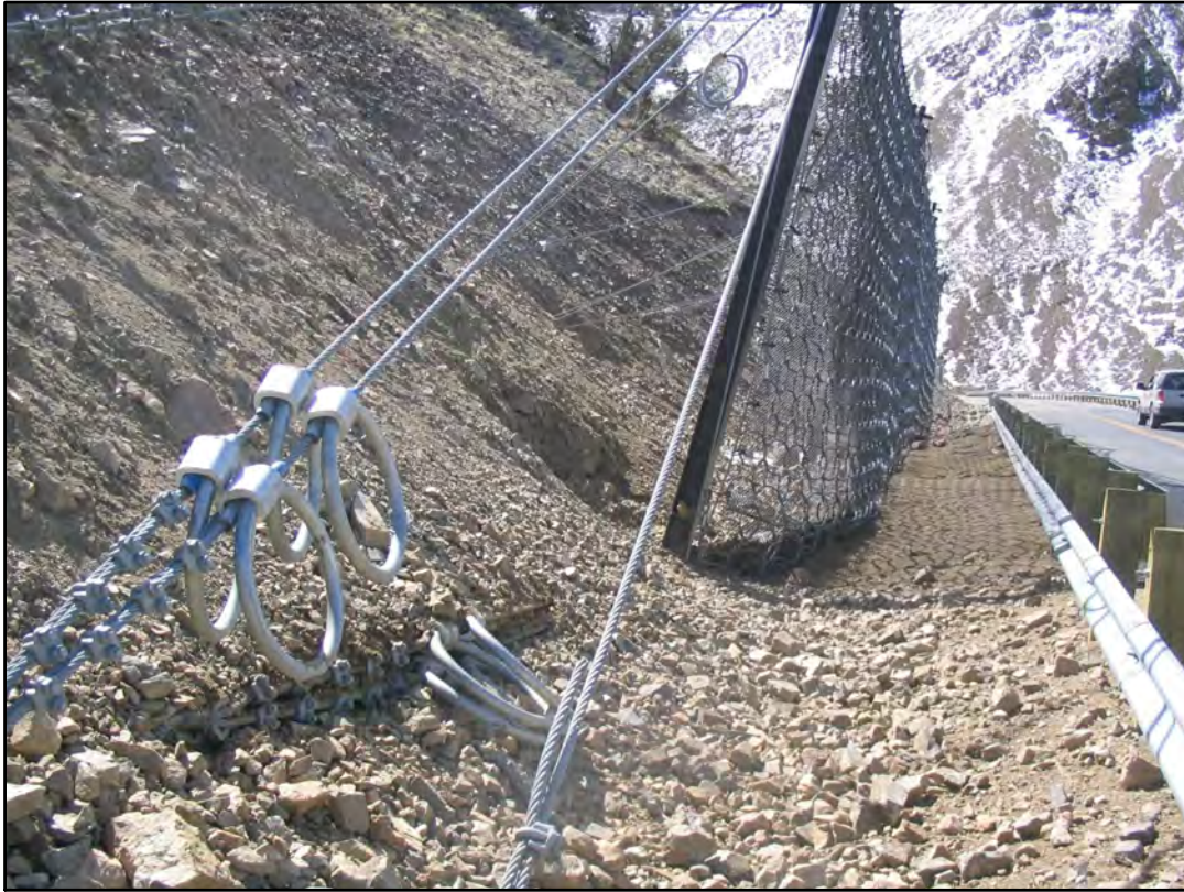
Photograph 17. Typical flexible debris flow barrier profile view. Beartooth Highway, 2005.
