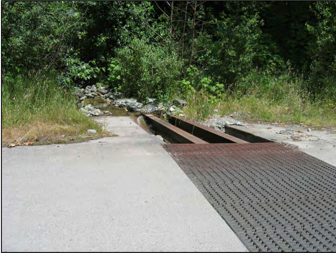
Photograph 19. Vented ford: close up of steel grate cover and trash rock.
