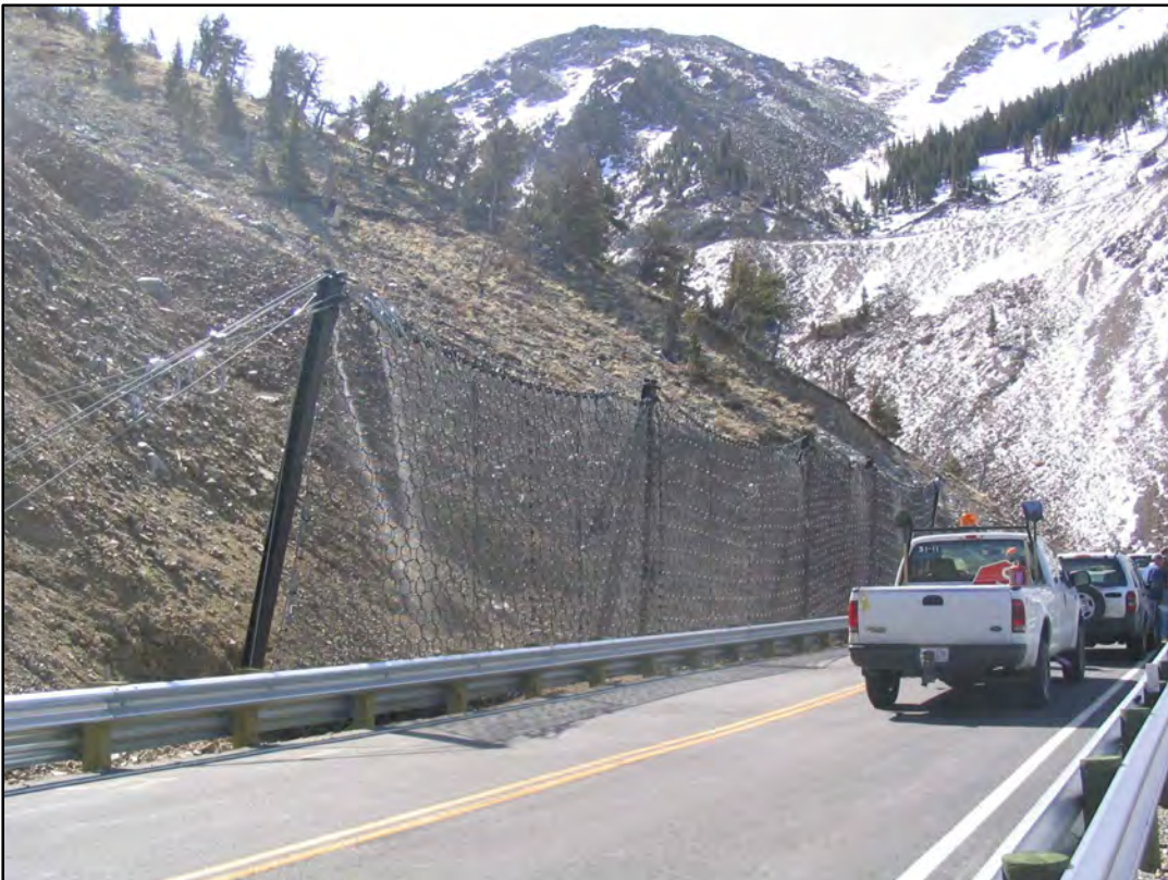
Photograph 16. Typical flexible debris flow barrier that was installed along the Beartooth Highway, MT, in 2005.
